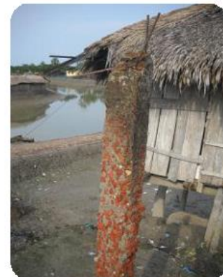
Erosion on walls and columns
